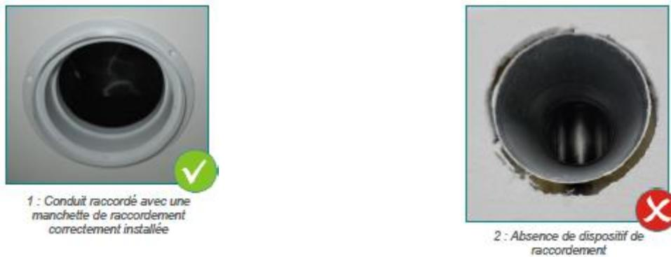
Figure 17 : Dispositif de raccordement bouche/gaine (Promevent)
